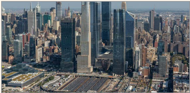
FIGURE 21. A view of Hudson Yards, NYC. The rail tracks are visible going under the completed half of the development.
